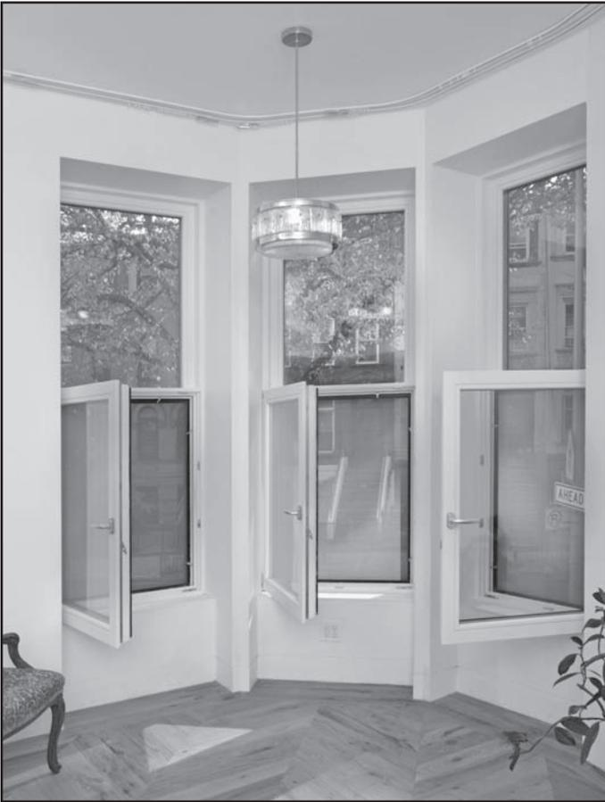
Figure 11. The new Zola American Heritage SDH™ is designed to aid historic properties pursuing energy-efficient restorations and high performance retrofits. Interior shot of the Zola Tilt & Turn simulated double hung design. Photo courtesy Teresa Peterson and Zola European Windows.
